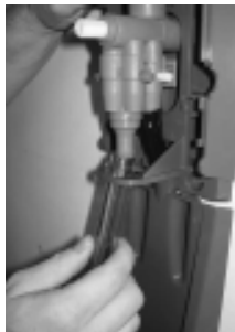
11. Install low flow (1.0 GPM) discharge tube.
